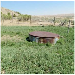
Note 1—Photograph shows a manhole-sized access leading to the well casing located in a field near a farm outbuilding. Releases of chemicals or petroleum products near or into a well can result in the contamination of the groundwater aquifer in which the well is constructed.
