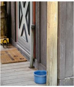
FIG. X1.9 Fill pipe for an underground storage tank containing fuel oil located on the back porch of a single family home.
