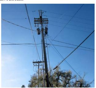
FIG. X1.3 Typical pole-mounted electrical transformers that may contain PCBs.
